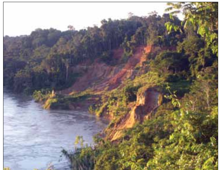
Fig. 7. Erosive bank of the Madre de Dios River near the CICRA station in Peru. Photo illustrates evidence of active mass wasting and a narrow segment of a fluvial terrace.
